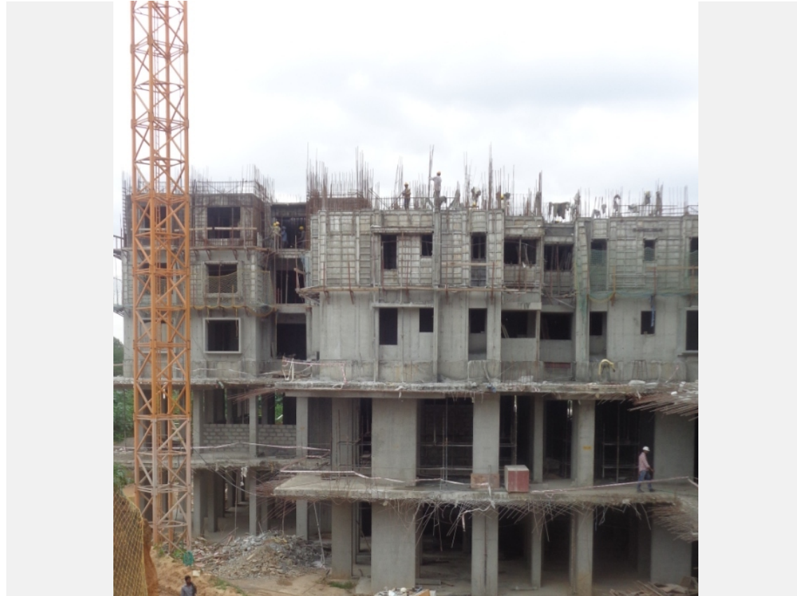
TOWER N Level 2 Roof Completed
