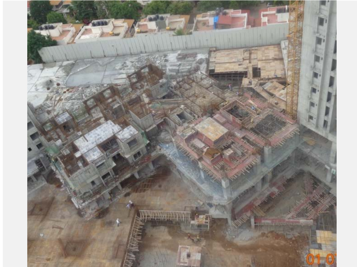
TOWER L Level 2 Work In Progress
